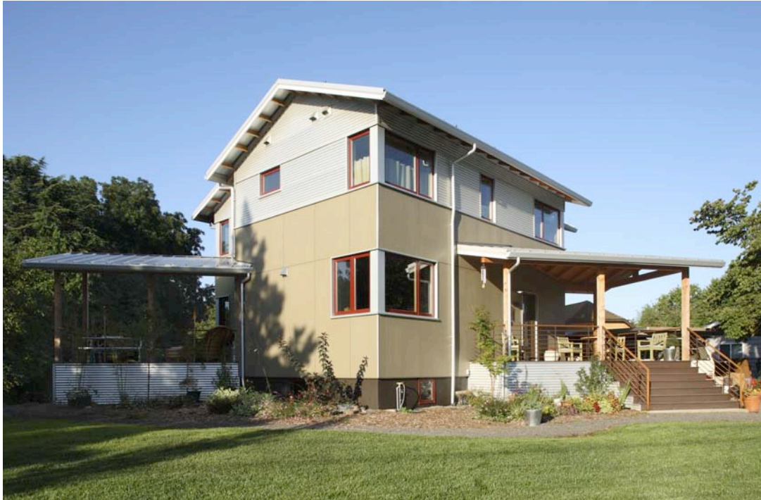
Passive Solar Design, Rain Screen, exterior foam to create thermal break
