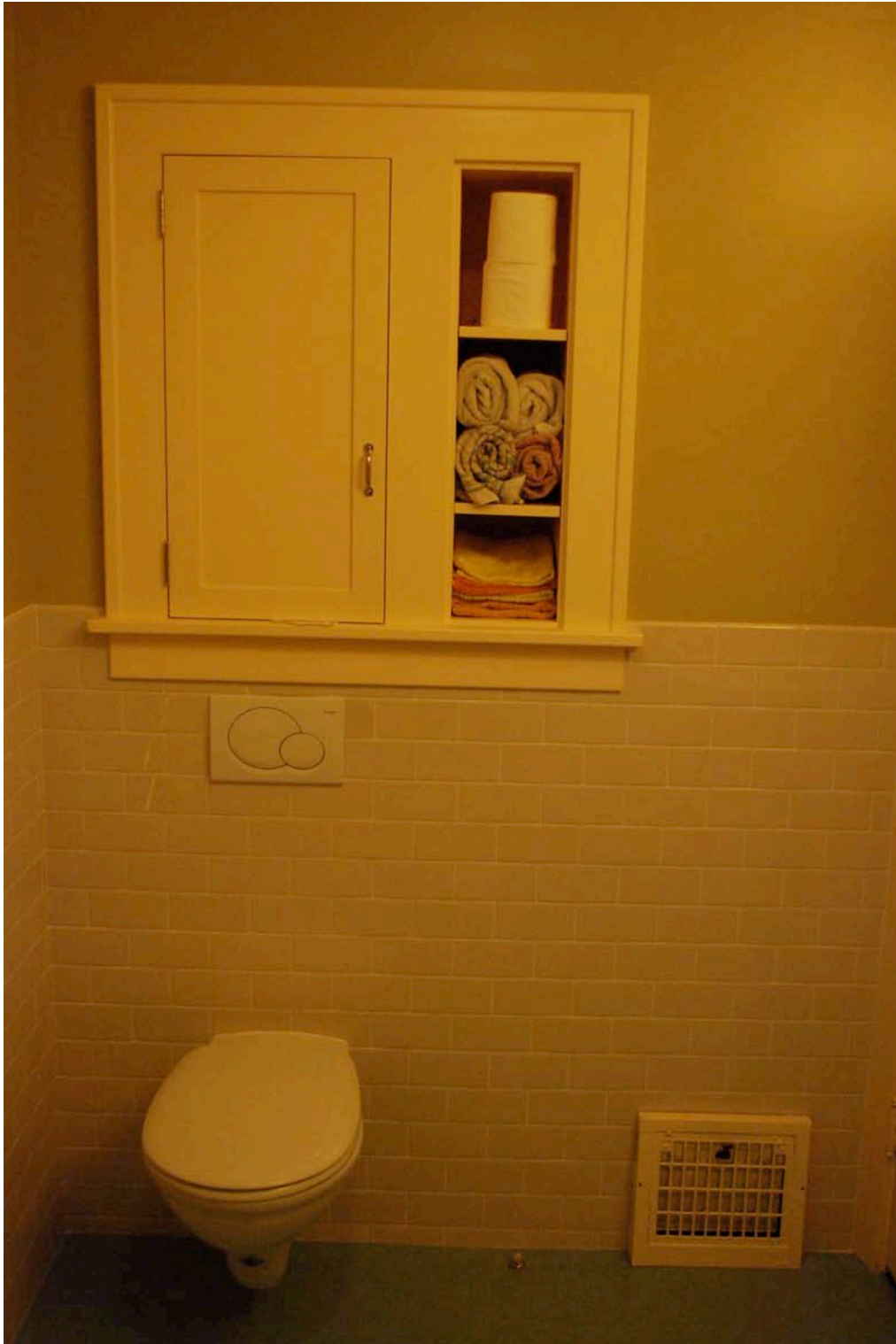
Wall mounted toilet to maximize space for aging in place, custom cabinet and towel organizer
