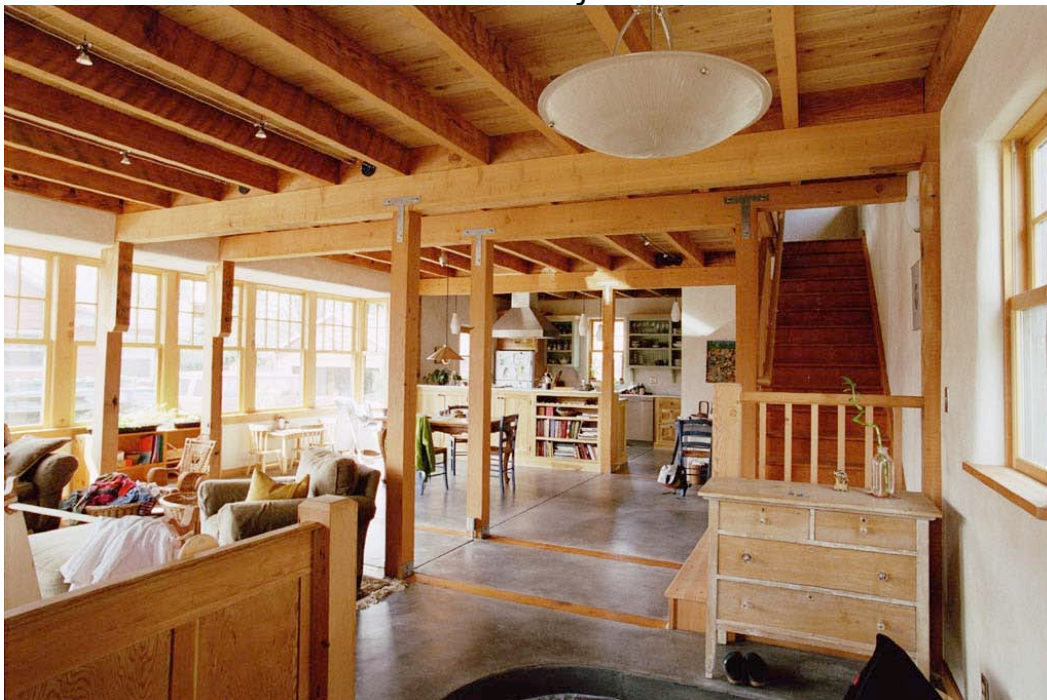
Radiant heated concrete floor; stair treads of reclaimed gymnasium flooring
