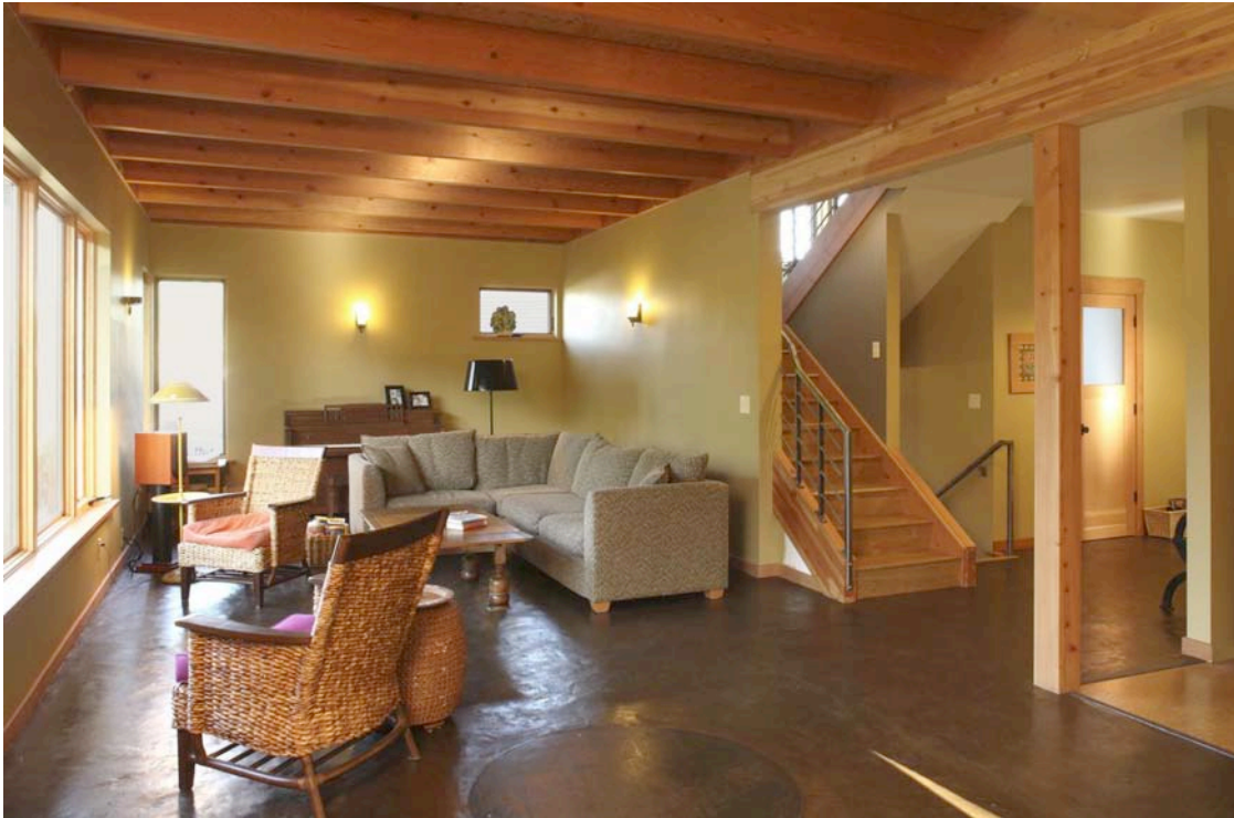
Exposed FSC beam ceiling, FSC OR white oak stair treads
