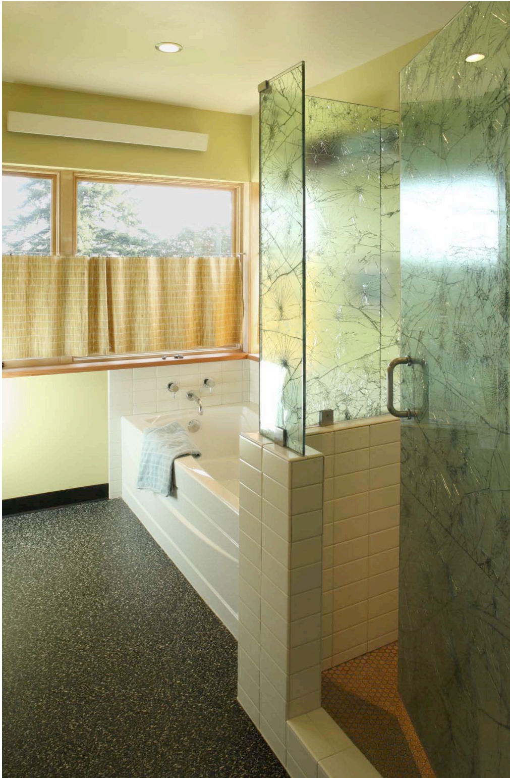
SecondGlass (reclaimed automobile windshields) shower enclosure in Master Bath
